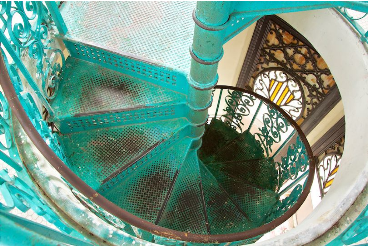
The staircase in Cienfuegos, Cuba, the "C" curve leads your eye downward. Note the presence of other geometric shapes as well; triangles, circles, ovals, and rectangles.
